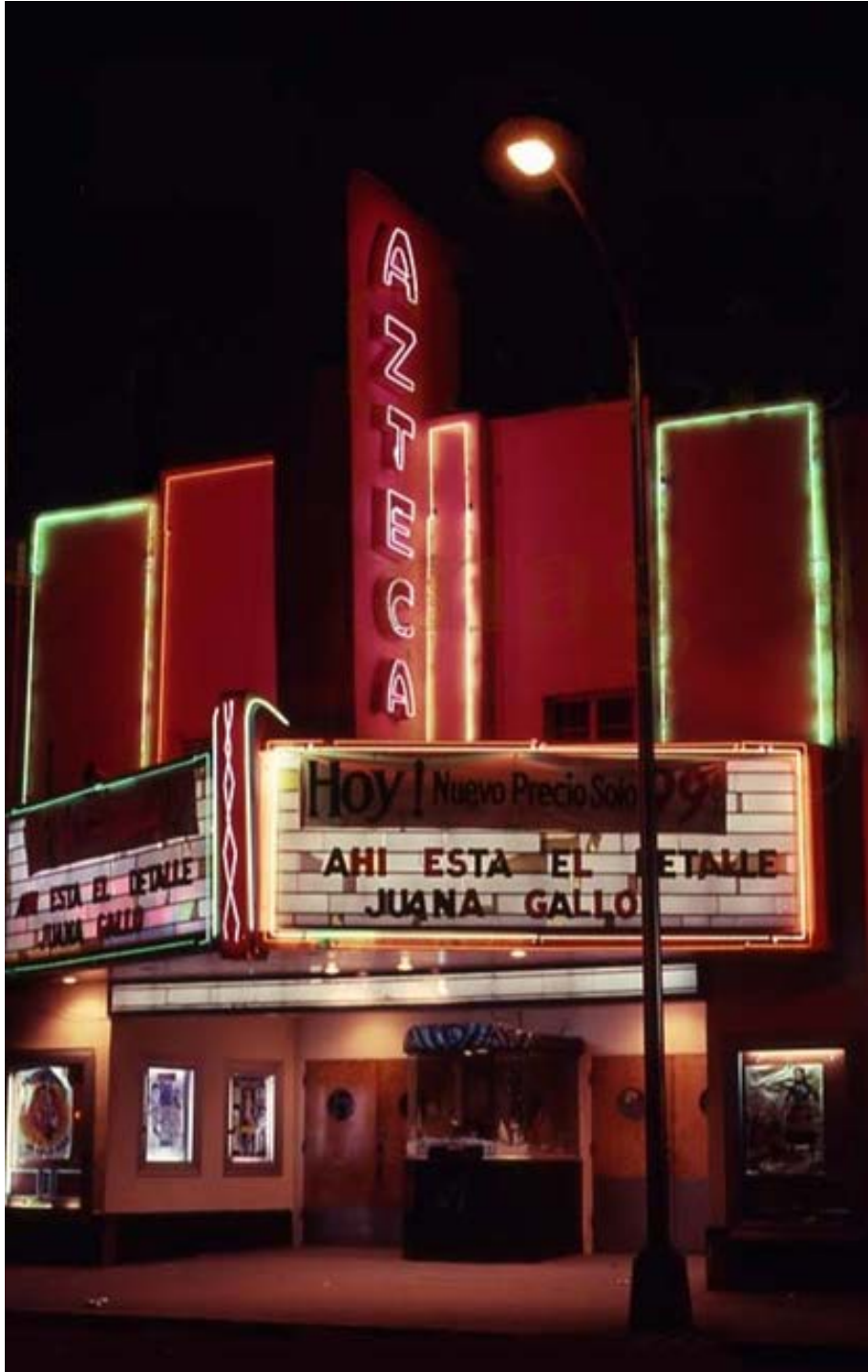
Figure 4. Primary façade, December 1982; Courtesy American Classic Images
